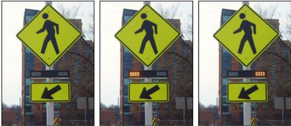
Figure 11 Rectangular Rapid Flashing Beacon
