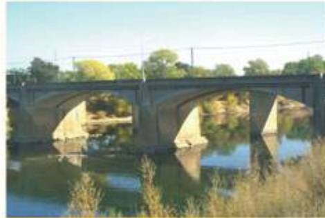
Del Paso State Route 160 Bridge
