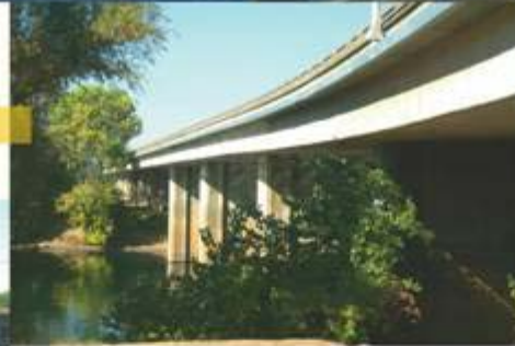
I-5 Bridge Over American River
