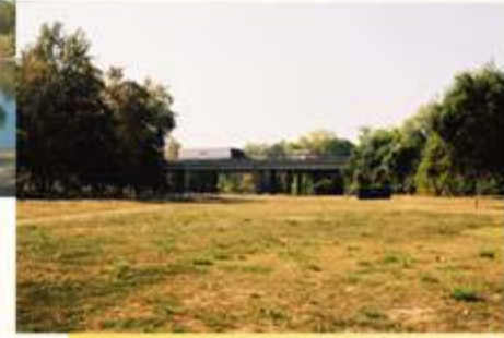
I-5 Bridge in American River Parkway
