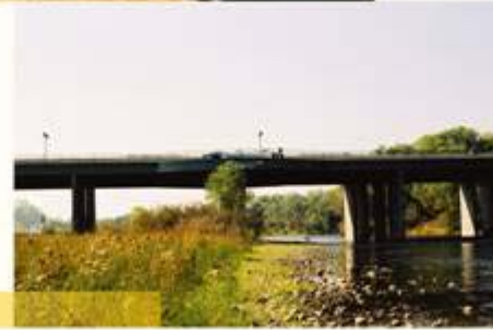
Watt Avenue Bridge Over American River
