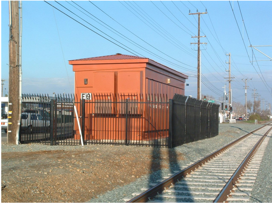
PLATE C-15: SUB-STATIONS TO RECEIVE AESTHETIC ENHANCEMENT
