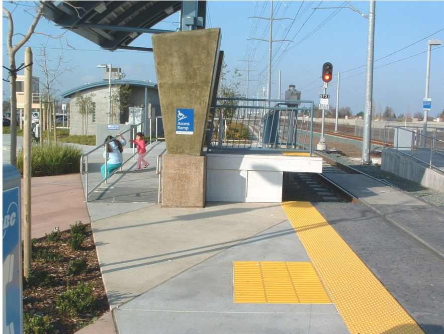
PLATE C-7: MINI-HIGH ACCESSIBLE RAMP
